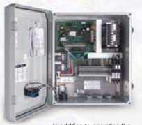
In addition to operating like other panels, the VeriComm Control Panel has four very "smart" functions: alarm management, data collection, troubleshooting, and advanced control logic. Operators can change settings at the panel from a PDA with Bluetooth<sup>®</sup>, or remotely via the web.
